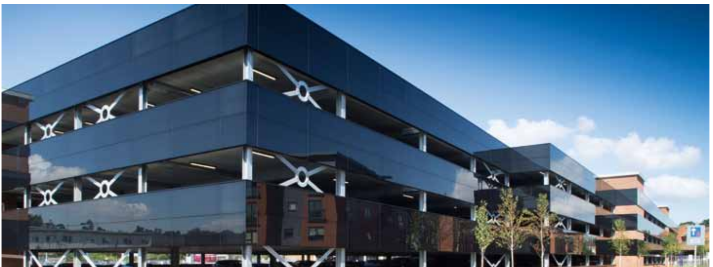
Exterior glass panel cladding installed by Berry Systems on the new Banbury railway station multi-storey car park. Berry also supplied and installed capping panels, soffits, internal perforated metal infill panels, link bridge security and access gate, rail side security mesh and their vehicle safety barriers, with anti-climb mesh and integral pedestrian handrail.
