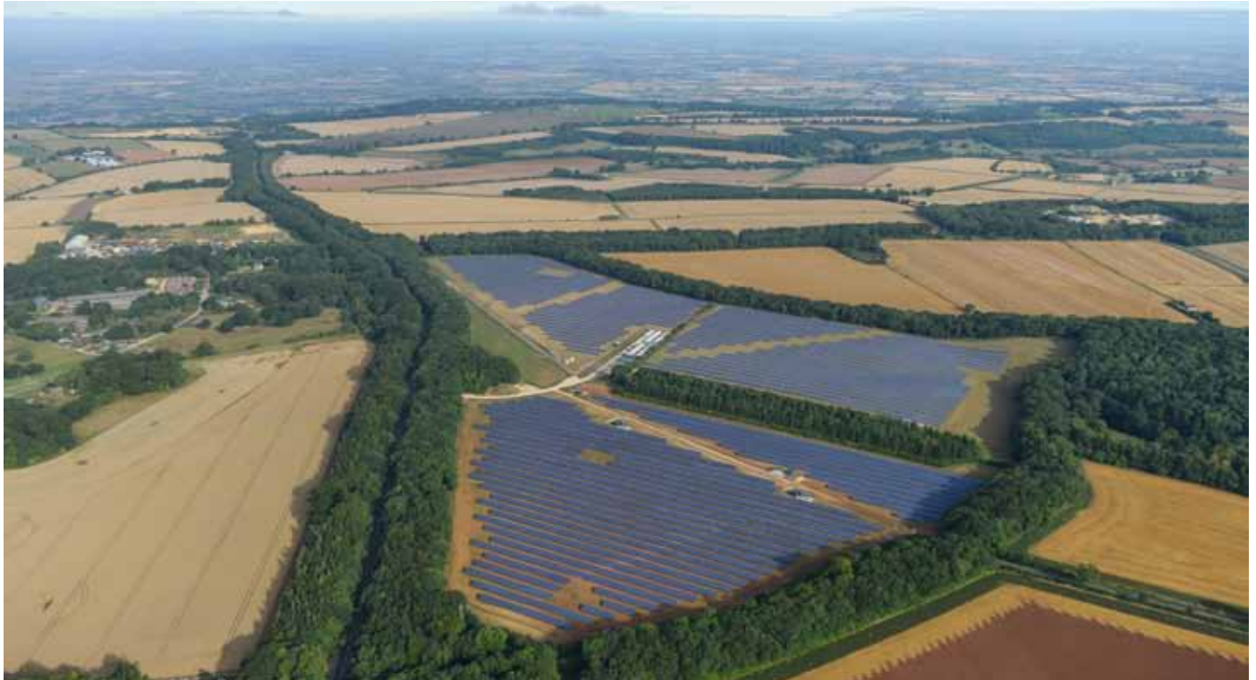
Hill & Smith Solar's 6.3MW/4 panel rows in a landscape orientation with a post driven foundation. The project is in the village of Blockley, a Cotswolds district of Gloucestershire, UK.
