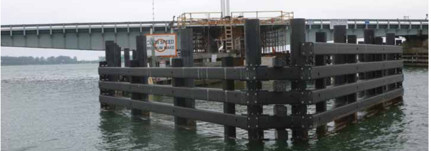
Creative Pultrusions supplied 113 GRP fender piles for the replacement of the Boca Grande North Swing Bridge Fender System in Florida, USA.
