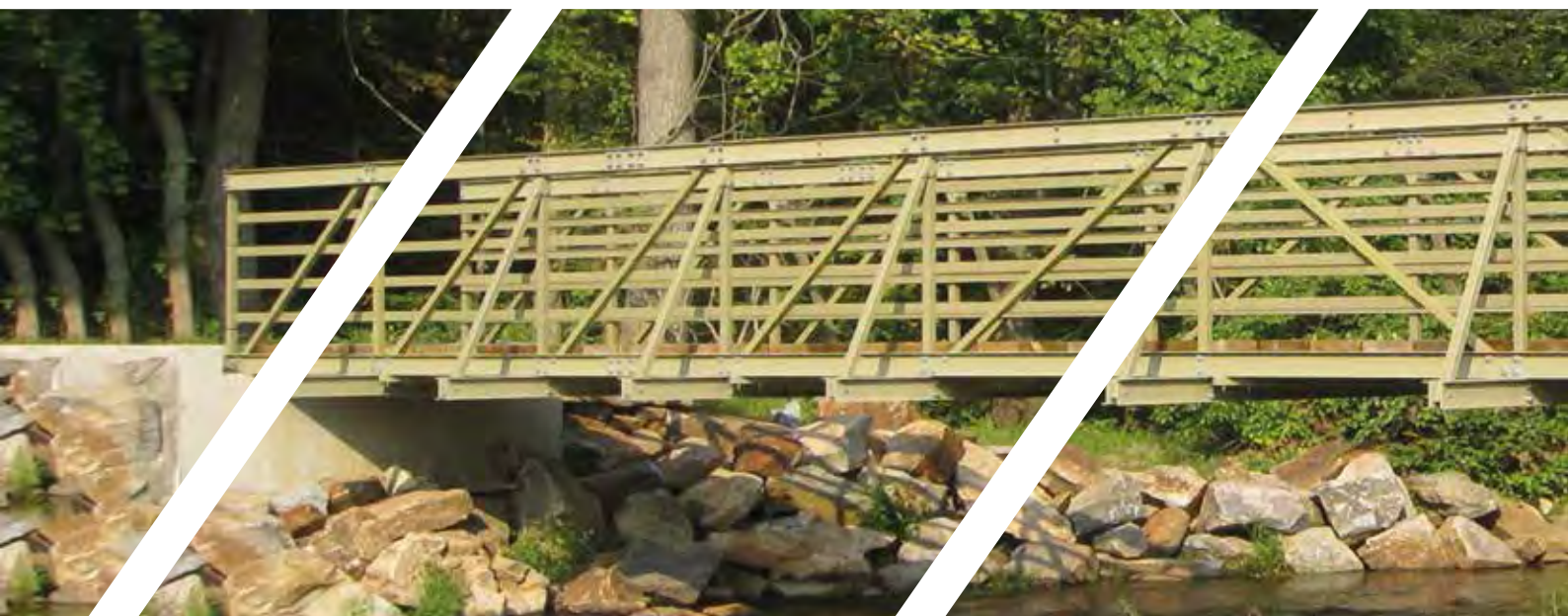
E.T. Technotics, Inc.'s composite bridge at Hopewell Dam - French Creek State Park, Pennsylvania, USA.
