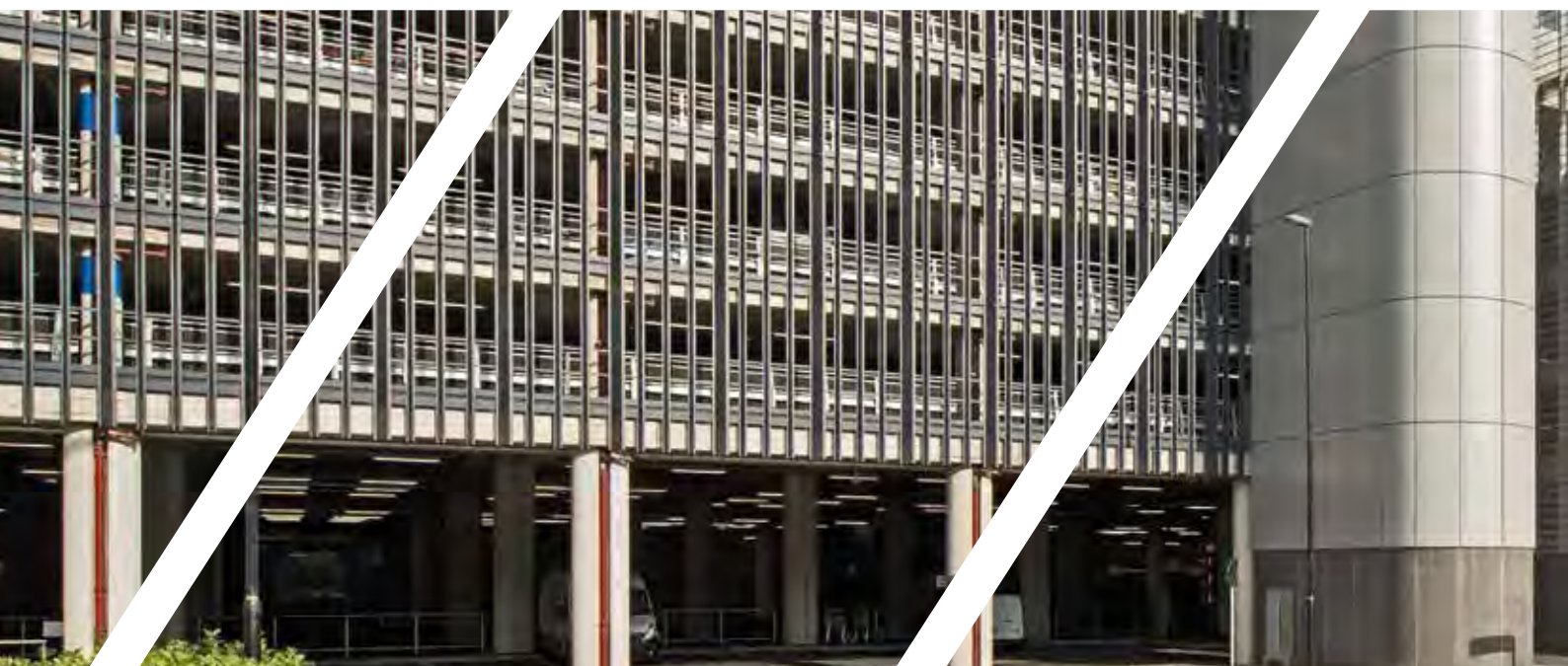
Perimeter and ramp barriers, installed by Berry Systems, for the new multi-storey car park at Terminal 2, London Heathrow Airport.
