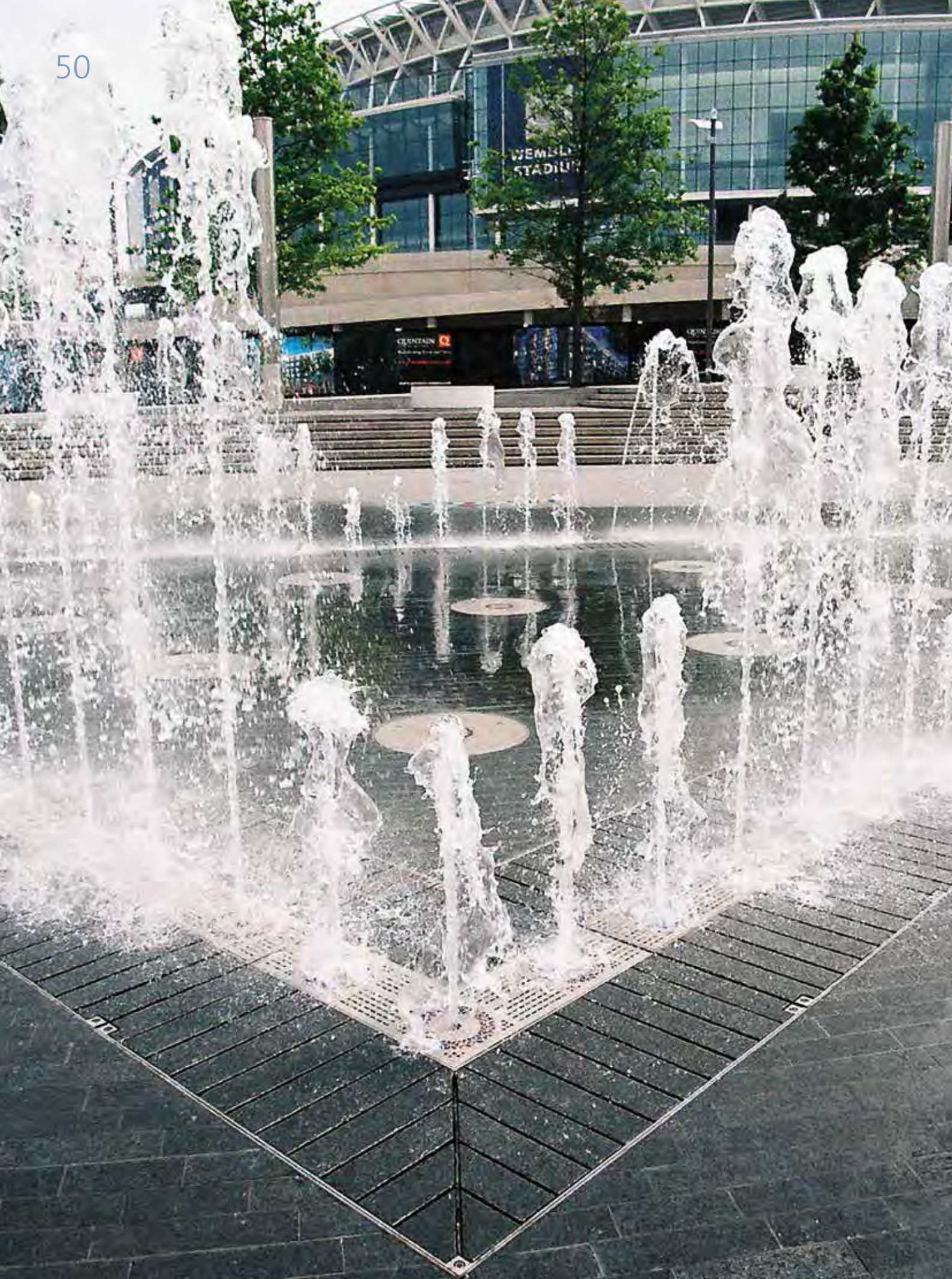
Jones of Oswestry's bespoke drainage, made from stainless steel and totalling 55m in length, creates a dynamic focal point to the landscape at Arena Square, Wembley.
